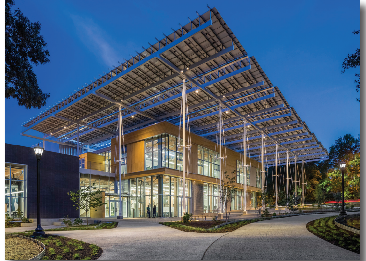
Kendeda Building for Innovative Sustainable Design at Georgia Tech, by Jonathan Hillyer.
