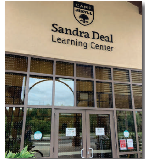
Bird-friendly film has been installed at Camp Jekyll thanks to a grant from the Disney Conservation Fund. Photo by Gabe Andrle.
